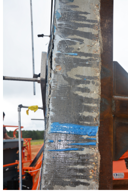
Figure 6: Concrete failure and debonding in FT1.
