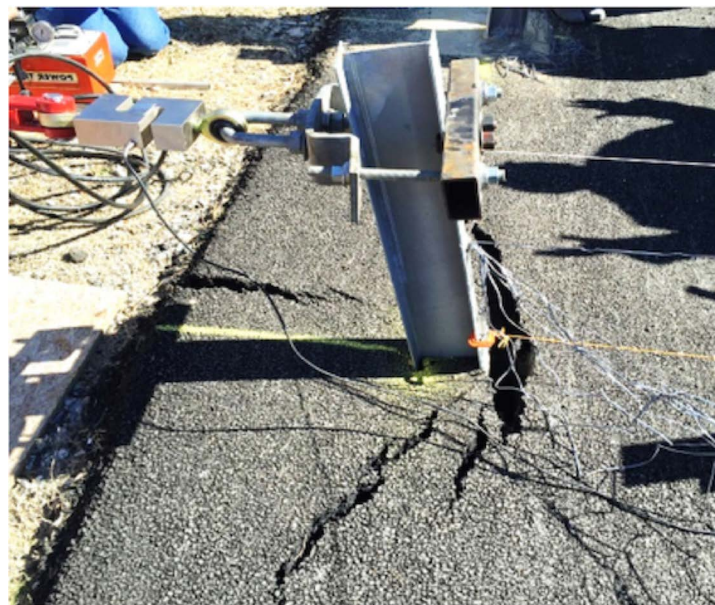
Figure 4. Asphalt rupture observed in the experimental program.
