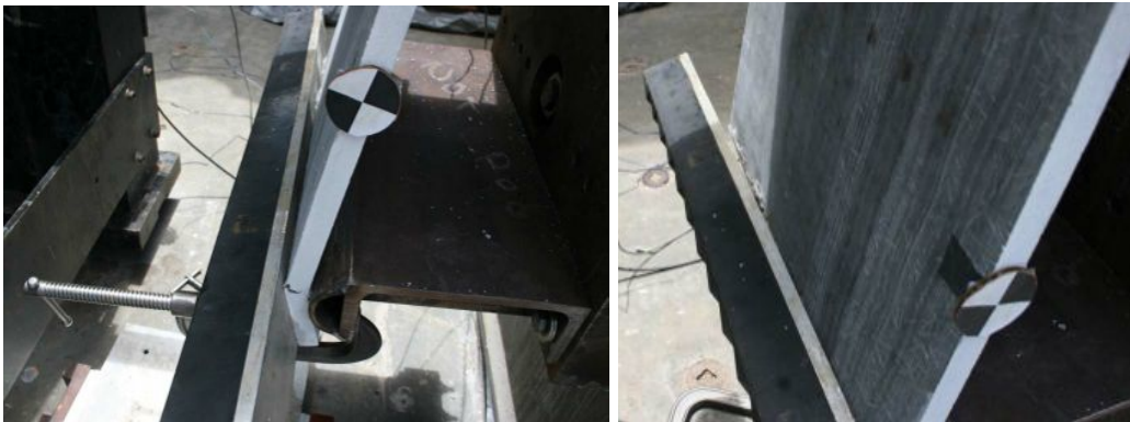
Figure 8: Test 7 posttest bottom connection damage.
