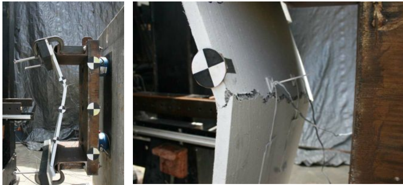
Figure 7: Test 7 posttest damage from side (left) and back (right).
